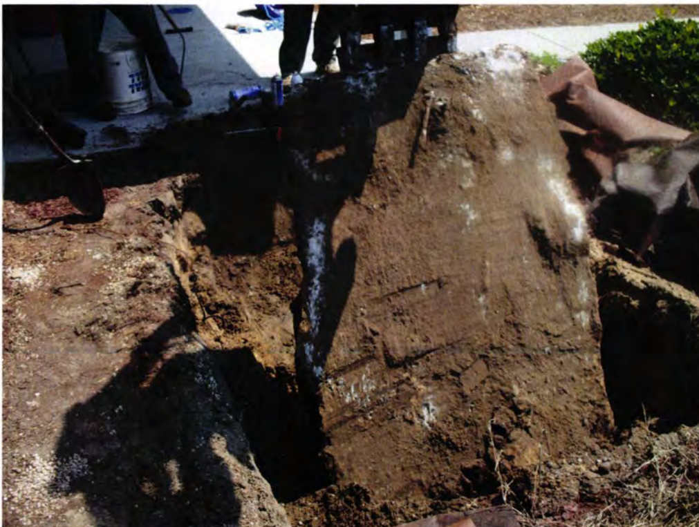
Picture 2: UST 320Ash excavation in progress.
